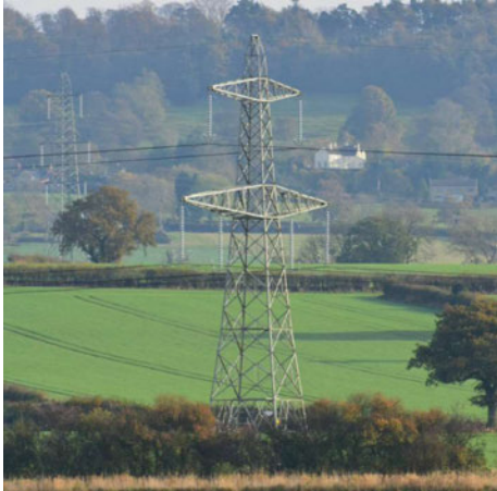
Image 4.3 - Typical low height lattice pylon
